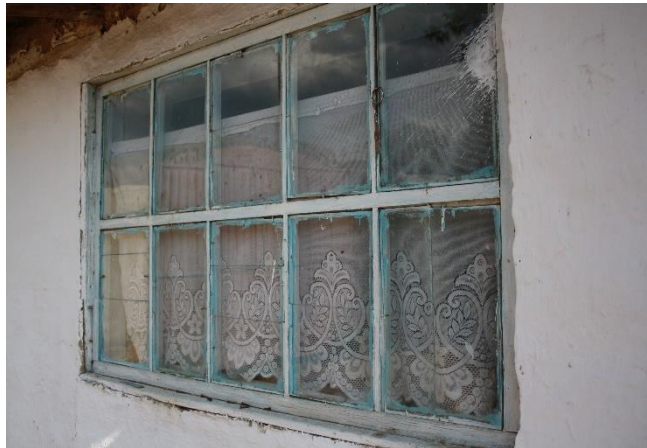
Figure 15: Window set directly into wall
