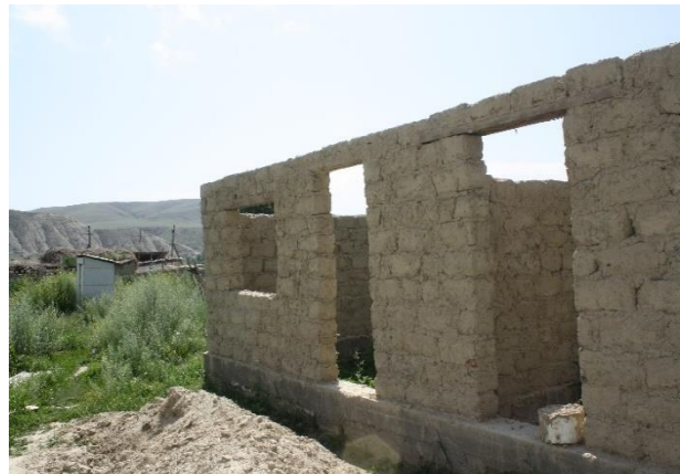
Figure 12: house being built
