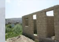
Stack 7: house being built
