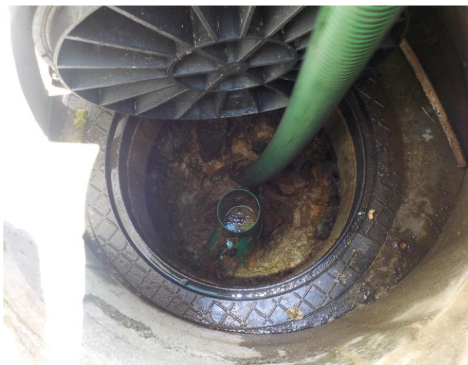
Figure 34: Pumping of scum in settler P1, August 14, 2018
