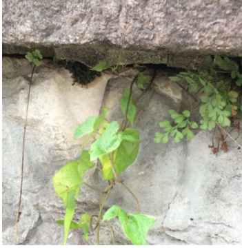
Figure 34 Example of plants with sprouting point on horizontal dihedral angle top on wall ID 18 (photo: S. Caregnato).
