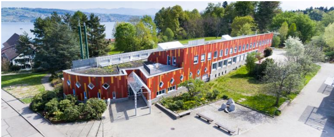
Figure 7 GA building, photo credit ZHAW
