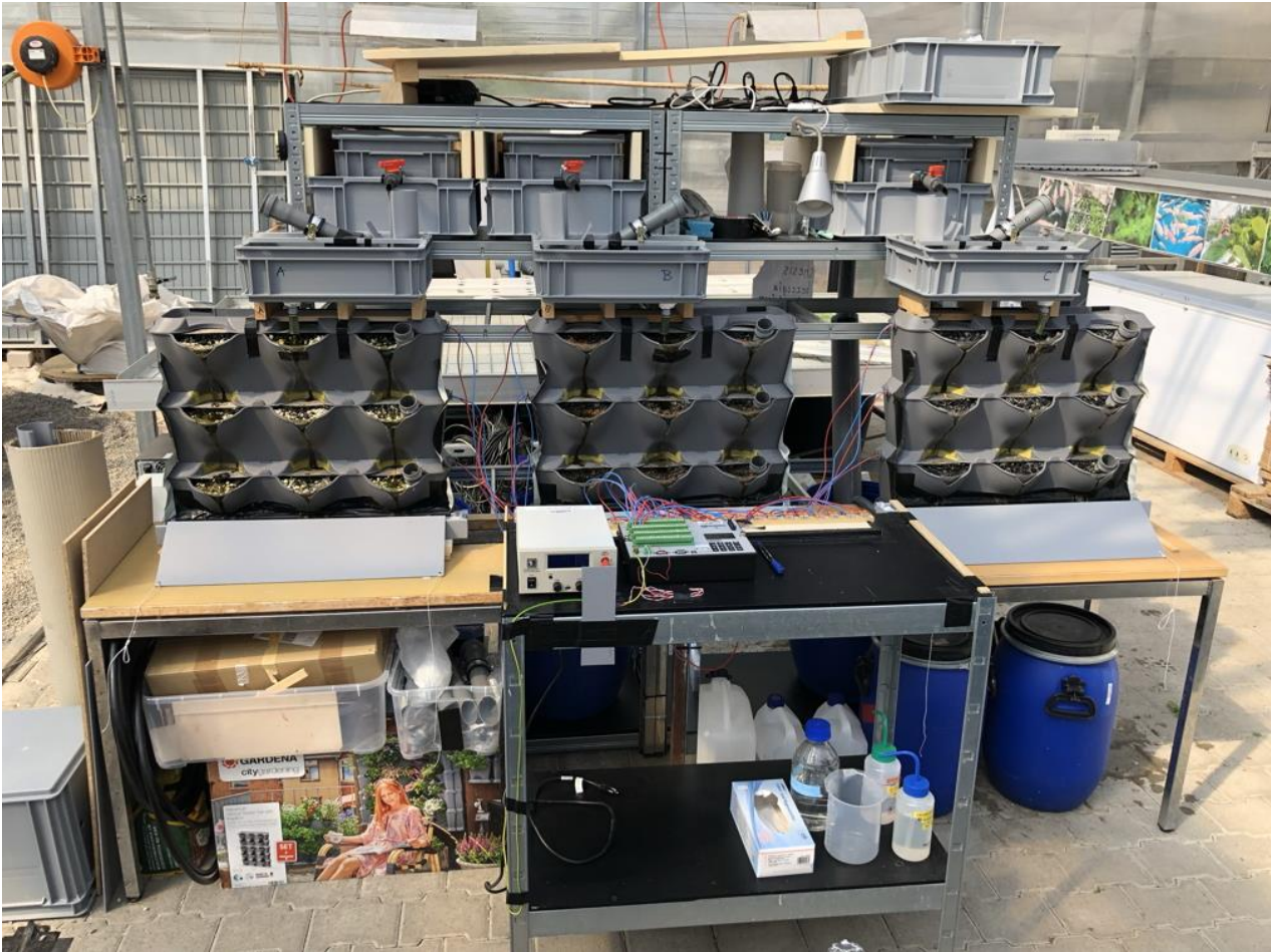
Figure 14: Overview of the experimental installation with the three systems. From top to bottom: head tanks, inlet pipes with regulation valve (orange), mechanical dosing apparatus, and the three green walls. From left to right: Wall A (Vulkaponic substrate), Wall B (Seramis expanded clay), and Wall C (HDPE biocarriers). On the table in the foreground: data logger.
