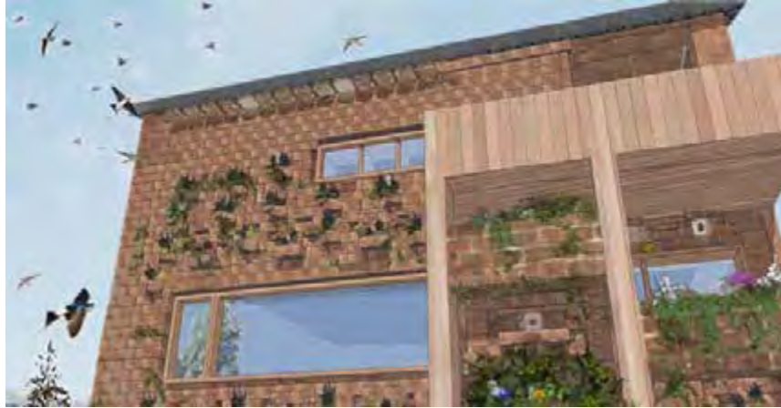
Figure 14: On the west-facing side, several brick beds are attached to columns so that larger plant species characteristic of the habitats Trifolion medii and Galio-Fagenion . are integrated into the building envelope. Among others: the blackberry ( Rubus fruticosus ), the hairy sedge ( Carex hirta ) and the spiky rapunzel ( Phyteuma spicatum ). The containers shade the facade behind them, which provides a semi-shaded and sheltered niche for the redstart. Plants of the Trifolion medii occur also in the modules near the balcony. On the upper edge of the facade, there are built-in structures on which house martins build their nests.
