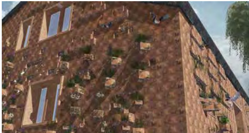
Figure 15: On the south-facing side of the facade, the habitat Centrantho-Parietarion is imitated. Apiaceae, such as the wild carrot (e.g. Daucus carota ), are planted to provide food for the masked bees. The spars in the modules can be used as summer roosts by smaller bat species such as the common pipistrelle. On the top floor, an entrance is built into the attic for the greater mouse-eared bat, separated from the space occupied by humans.
