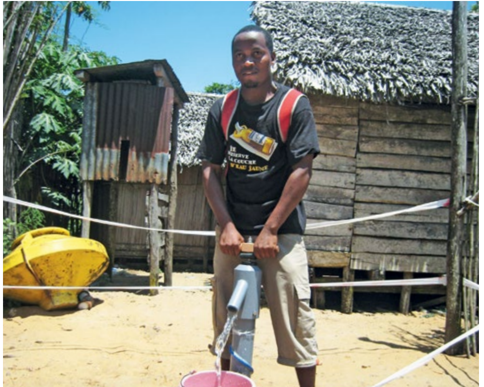
A Bushproof employee pumps water from a temporarily installed well. (All pictures by Martina Binder)
