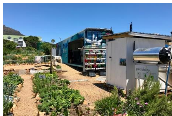
Figure 17: Expansion of the LaundReCycle with a shower and hydroponic system with the aim to explore wider greywater reuse applications
