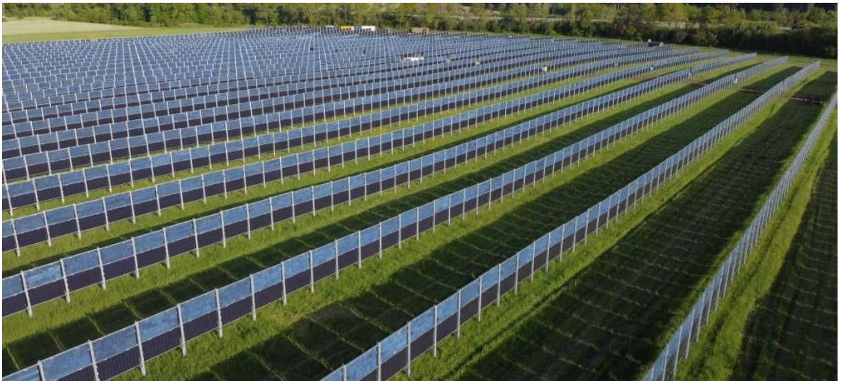
Figure 3: System example for the "permanent grassland" management status. Vertical APV system from Next2Sun in Donaueschingen (Germany). The bifacial modules are vertically elevated, orientation of the module surfaces to the east or west, row spacing 10 m (Next2Sun, 2020).
