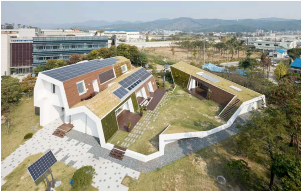
Figure 8. Aerial view of Kolon e+ Green Home. Well visible are the greened roof, facades, roof-integrated PV generators and solar thermal collectors. The Kolon headquarter building is visible in the background left.
